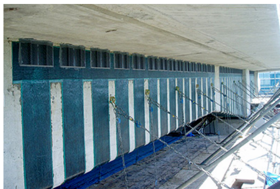
Genta Bridge under construction
