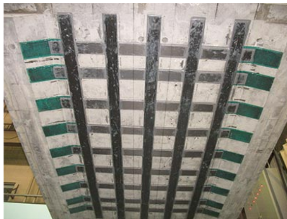
Deck slab reinforced with e-Plate
