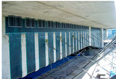
Genta Bridge under construction
