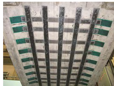
Deck slab reinforced with e-Plate
