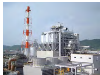
Biomass boiler at the Hiroshima Plant
