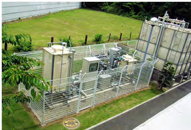
Decentralized water treatment & supply system
