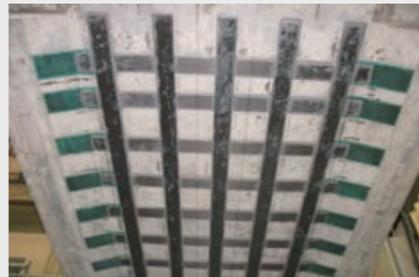
Deck slab reinforced with e-Plate
